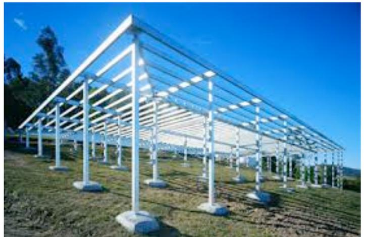
*Lightweight steel floor frames are inherently resonant*
