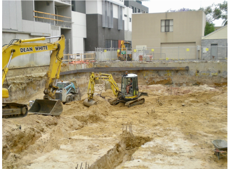
Major excavations close to other buildings can be a challenge
